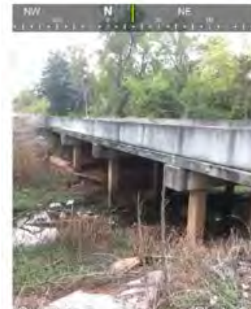
FIGURE 13: UPSTREAM FACE OF BRIDGE
