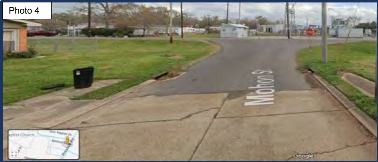
Street view of the roadway drainage in the area – Mohon Street.
