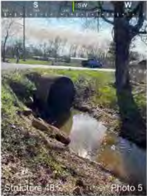
FIGURE 7: UPSTREAM VIEW OF CULVERT
