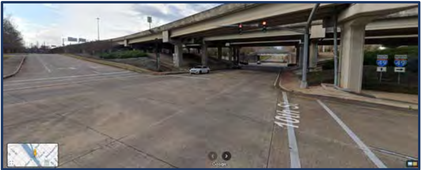
Google earth view of the clearance and grade under the bridge.
