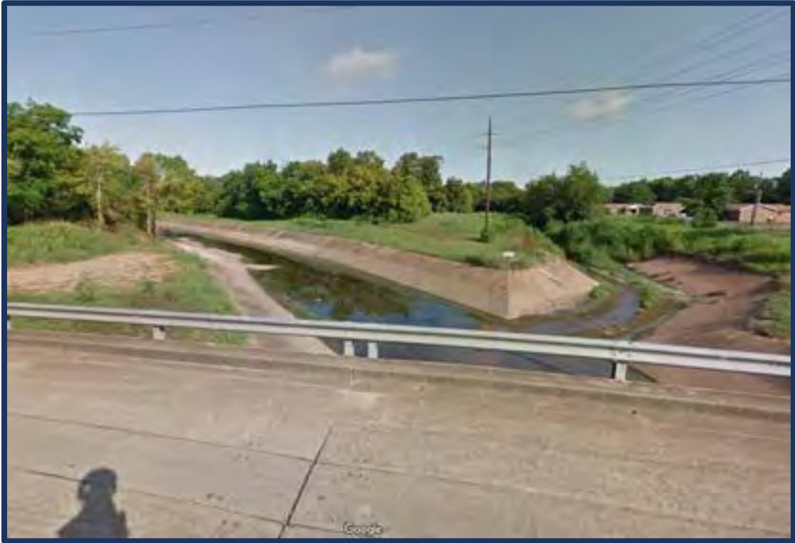
Northwest street view of the hardened portion of the Horseshoe Drainage Canal from Tulane Avenue.
