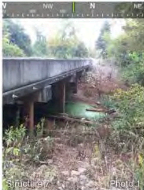
FIGURE 9: DOWNSTREAM FACE OF BRIDGE
