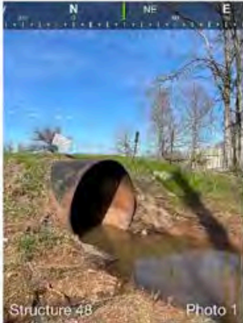
FIGURE 3: DOWNSTREAM FACE OF CULVERT
