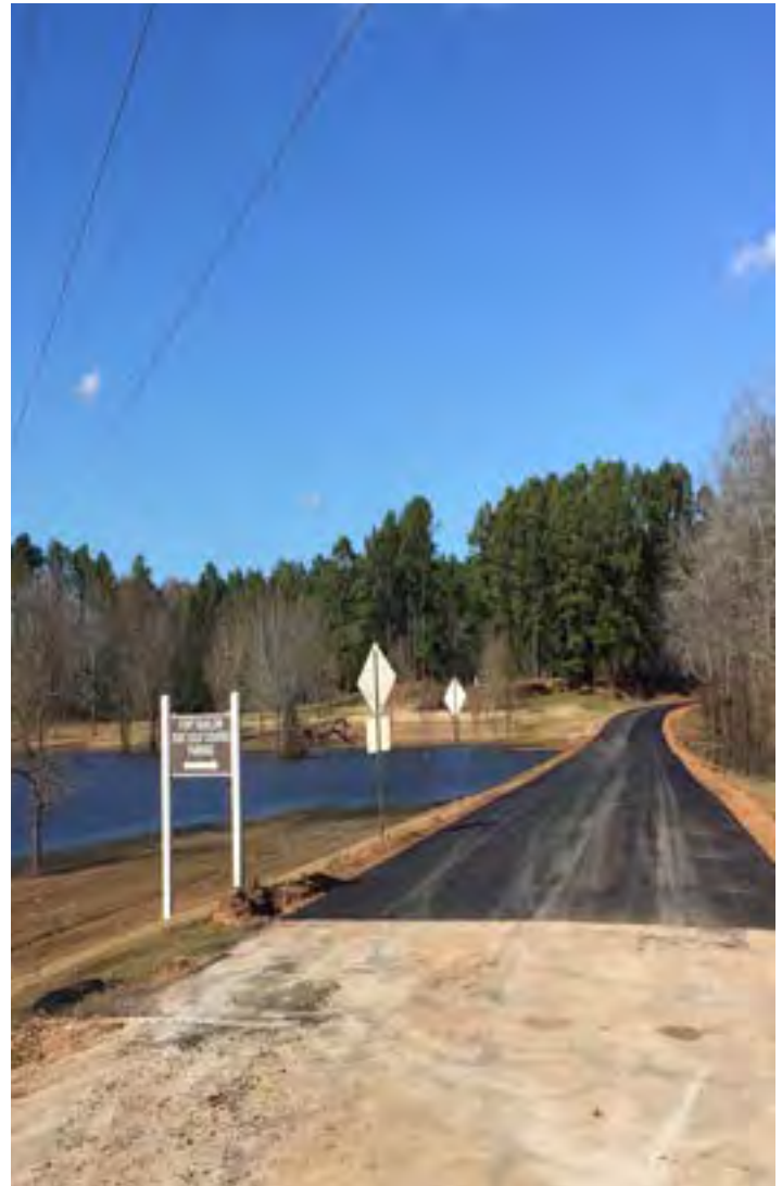
Photo 10.0: Roadway Construction at Buhlow Lake Pineville, LA
