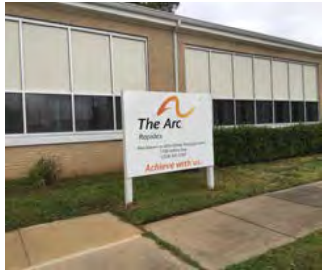
Photo 6.2: Human Service Transit Facilities
