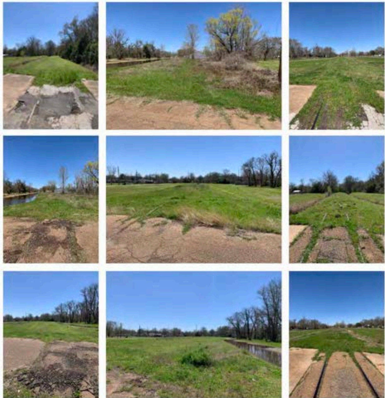
Figure 5A | MoPAC Rail Bed Inactive Segment (North of I-49)
