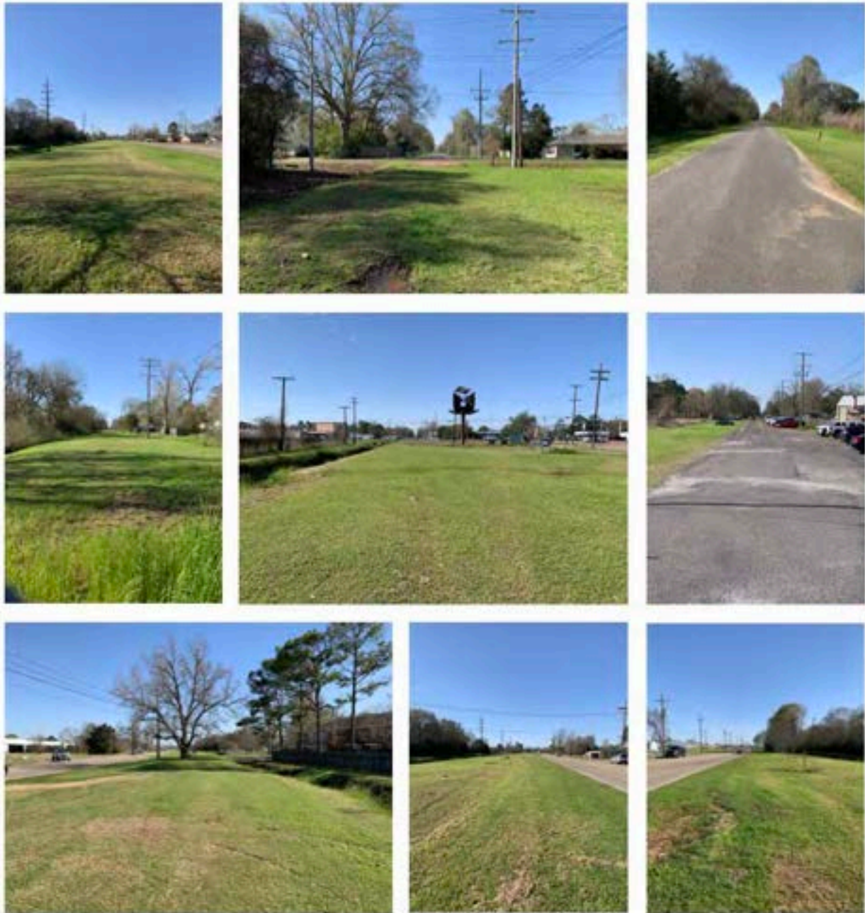
Figure 6A | MoPAC Rail Bed Inactive Segment (South of I-49)
