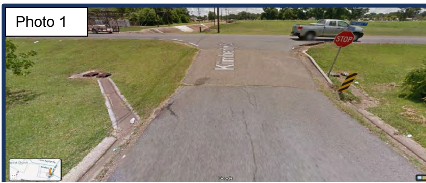
Street view of drainage in the area - Kimberly Street.
